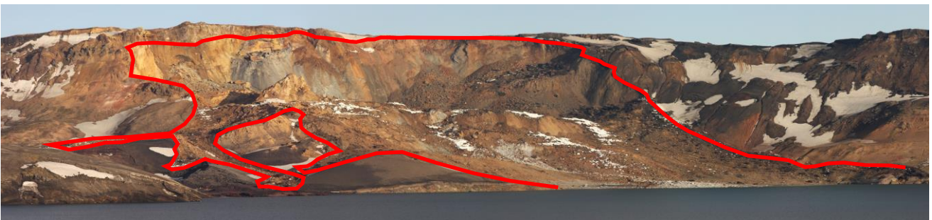
Figure 2. A photograph taken three days after the rockslide. The outline of the slide is indicated in the picture. Photo and drawing: Jón Kristinn Helgason, 24.7.2014.
